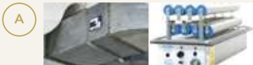
AtmosAir Bipolar Ionization Generator inside supply air duct.
