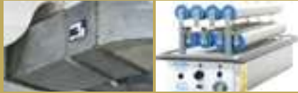
AtmosAir Bipolar Ionization Generator inside supply air duct.
